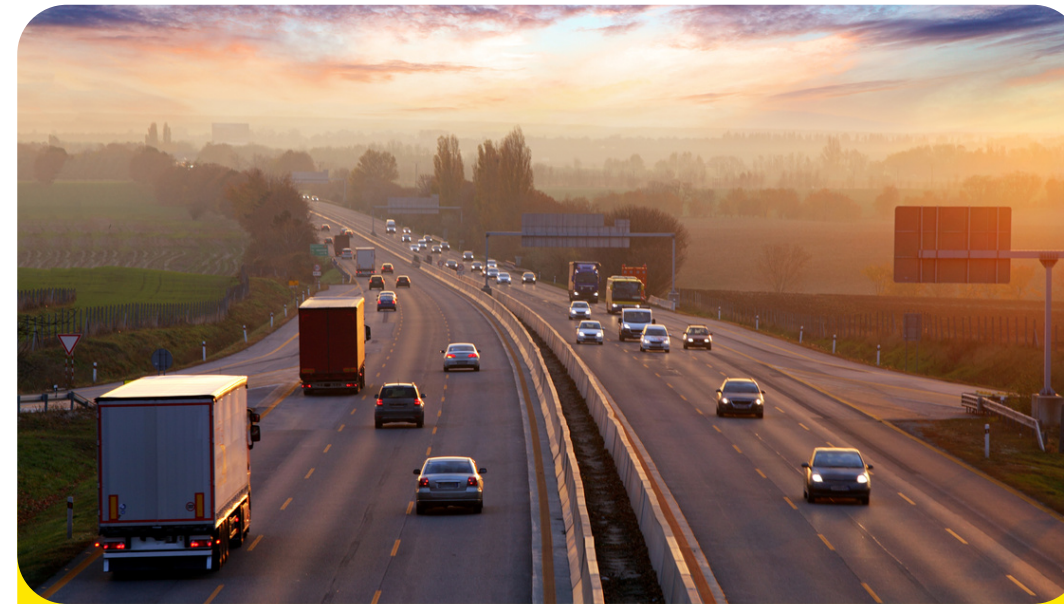
6 lane 200 feet radial road road
